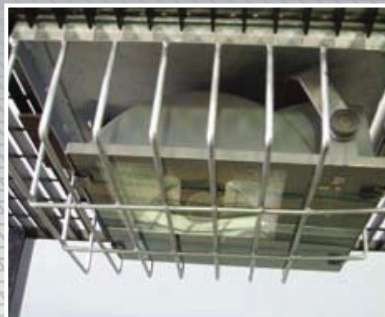
The Light Hatch is closed after the lamp is changed. The handle is pushed back into place and the walkway returns to normal.
